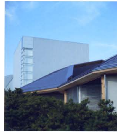
Joint between the two roofs
