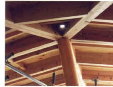
Top of column at roof joint
