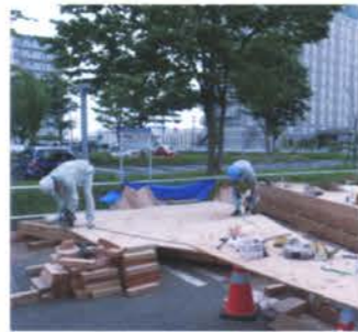
Top: Construction photos of roof from above and below
